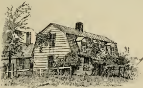
CORNER BRIDGE STREET AND LINCOLN AVENUE
